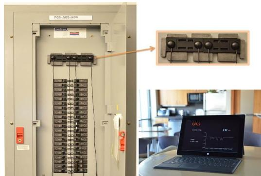
**Figure 1: Left: Contactless power consumption sensor on the breaker panel; Right: An interface showing whole-home total power consumption in real-time.**
